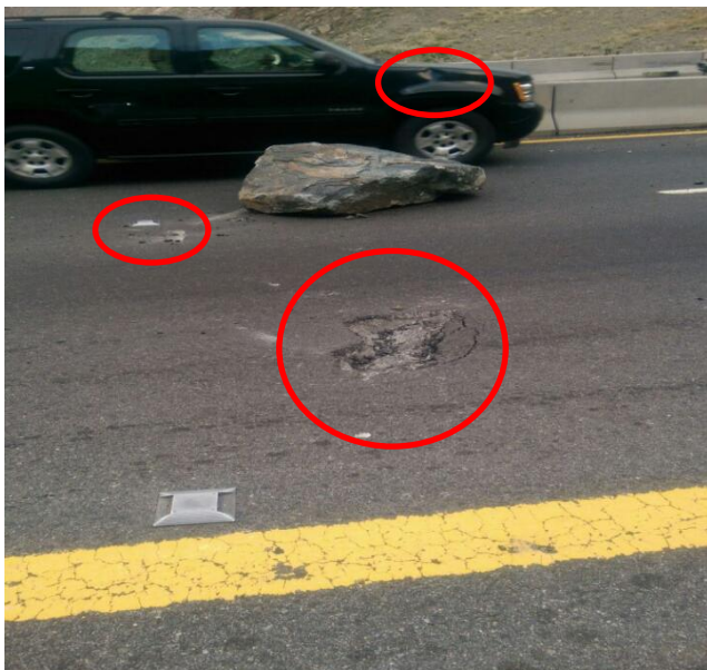
Fig. 6. A fallen rock block hit a car in the ascending road
