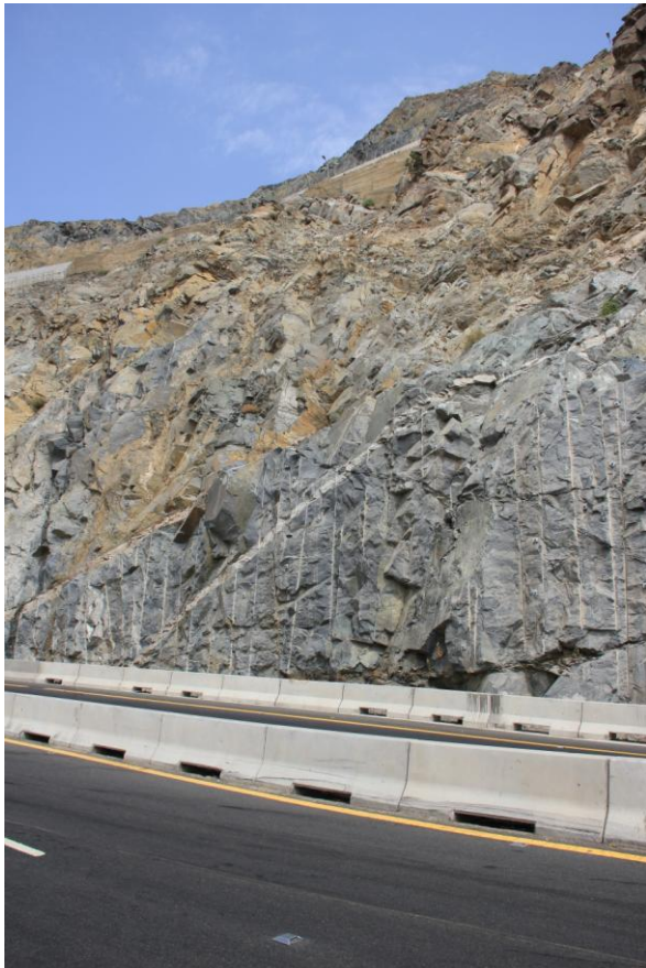
Fig. 4 Man-Made and Natural Rock Slope Along the Road.
