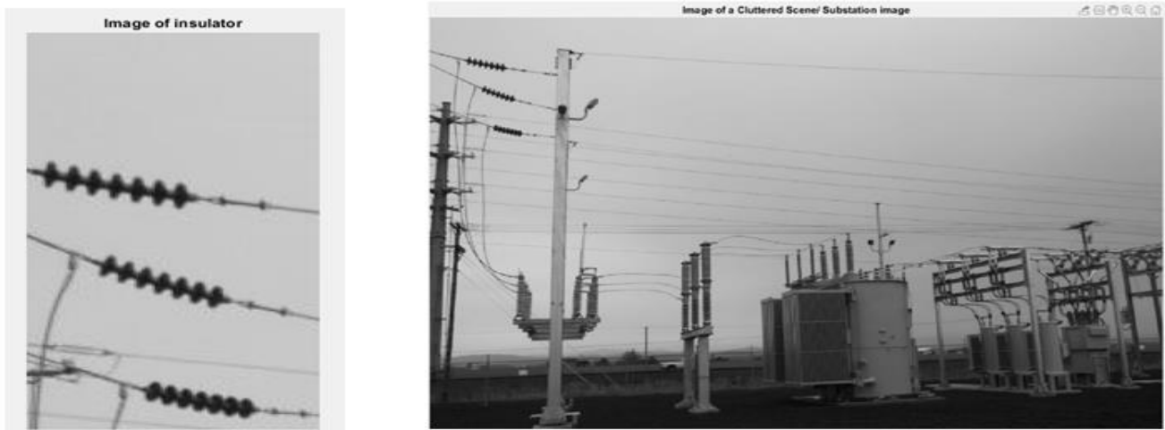
Fig. 7 Image of insulator/ Reference image Fig. 8 Image of a cluttered scene/ Substation image
